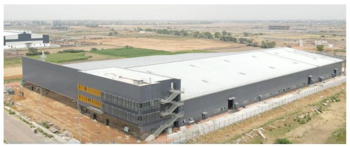
Another design highlight of this building is Hanging Staircase. The connections are made in such a way that even without columns this staircase has zero vibration. The connections have octagonal joints which helped to deliver this specialised staircase.
